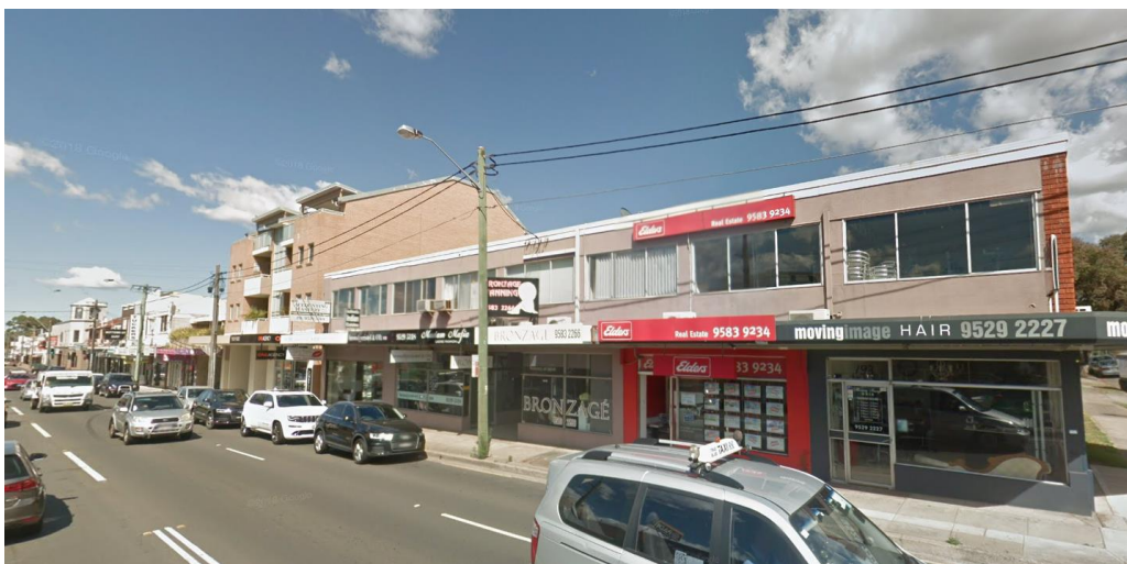
Figure 6 – 193-201 Rocky Point Road, Ramsgate (Source: Google Maps street view).
